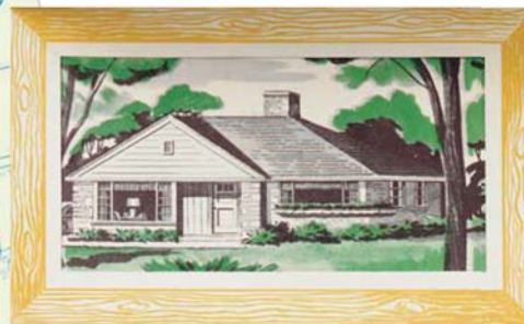
Chicago's COMPLETELY PLANNED Suburb
